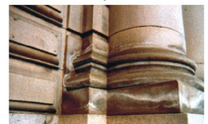
Efflorescence
